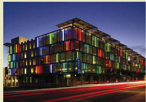
City of Santa Monica parking facility
