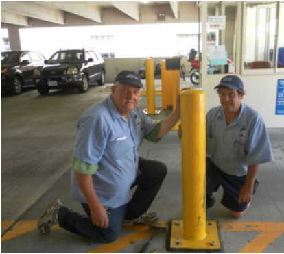
Clay and Stefon repair a bollard.
