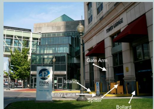
While all these terms are equally relevant in the parking industry, the term Access and Revenue Control "ARC" is one of the most important. Access and revenue control systems allow parking operators to identify the vehicle and record the time of entry. These systems can speed entry and exit from a facility and provide secure revenues and also alert the operator that a gate is malfunctioning.
